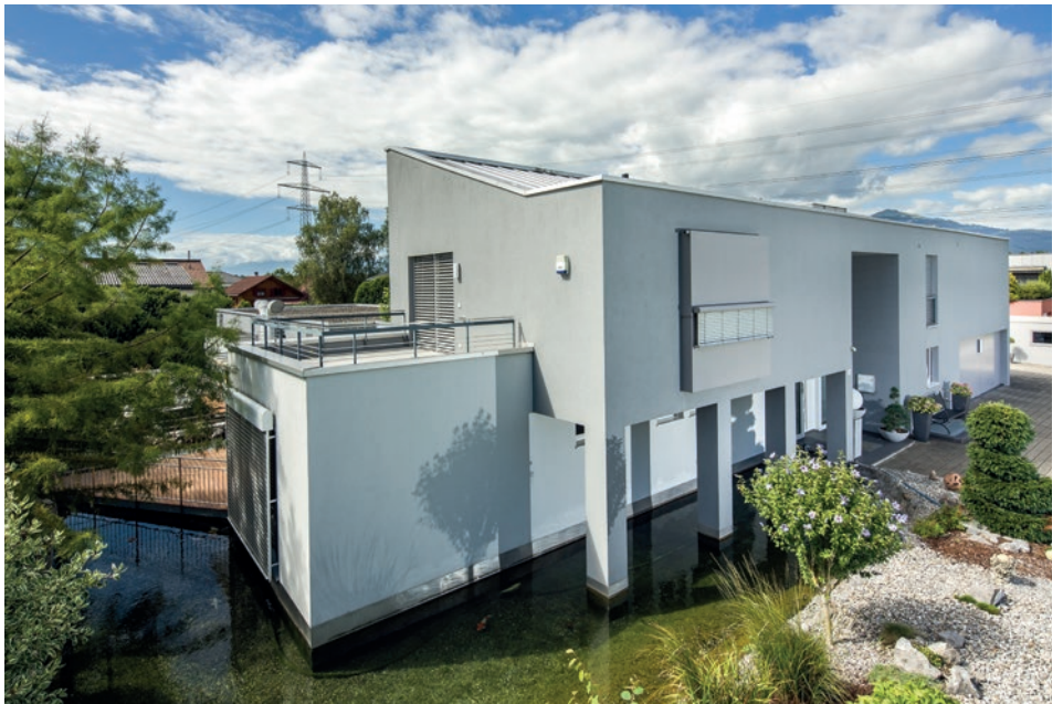
Roofinox Plus, double lock standing seam, private house A, Vorarlberg, Austria
