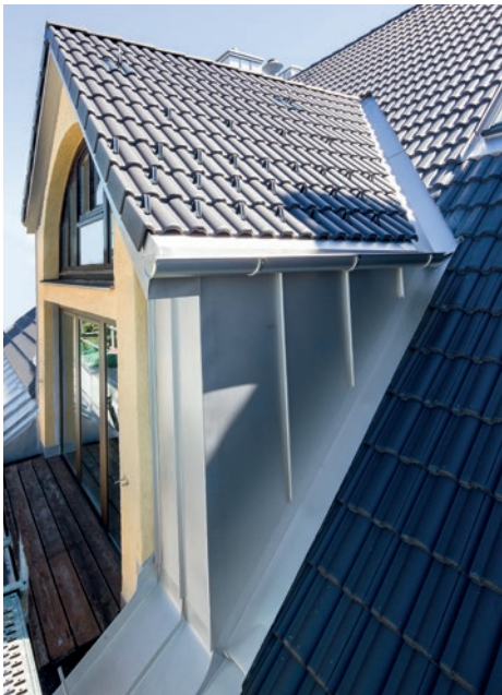
Roofinox Classic, dormer cladding and drainage, duplex, Munich, Deutschland
