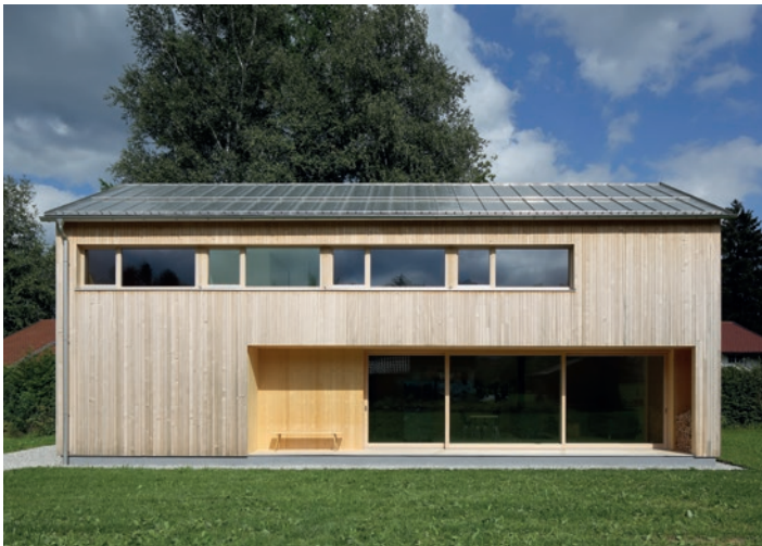
Roofinox Tin, double lock standing seam, private house B, Bad Kohlgrub, Germany
