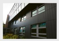
Reveal Panels can be produced in Copper, Brass, Bronze, Zinc, Stainless Steel, Precoated Aluminium and GreenCoat steel as well as powder coated Aluminium and Anodised Aluminium.
