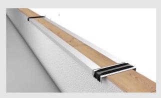
Lay the breathable metal separating membrane between the connectors, over the fixing strips.
